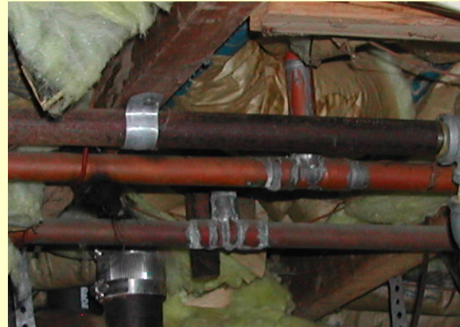
Uninsulated pipes in two PV homes
