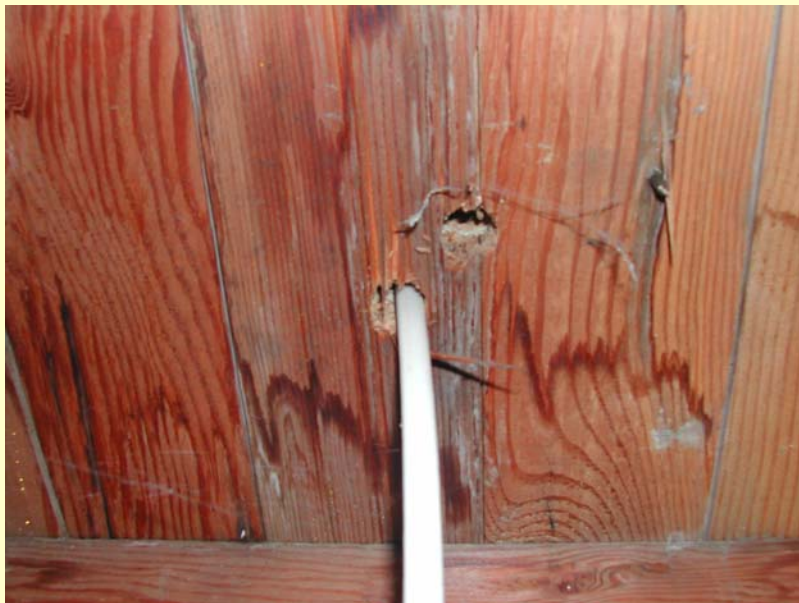
Holes around wire and pipe penetrations from crawl space in 2 PV homes
