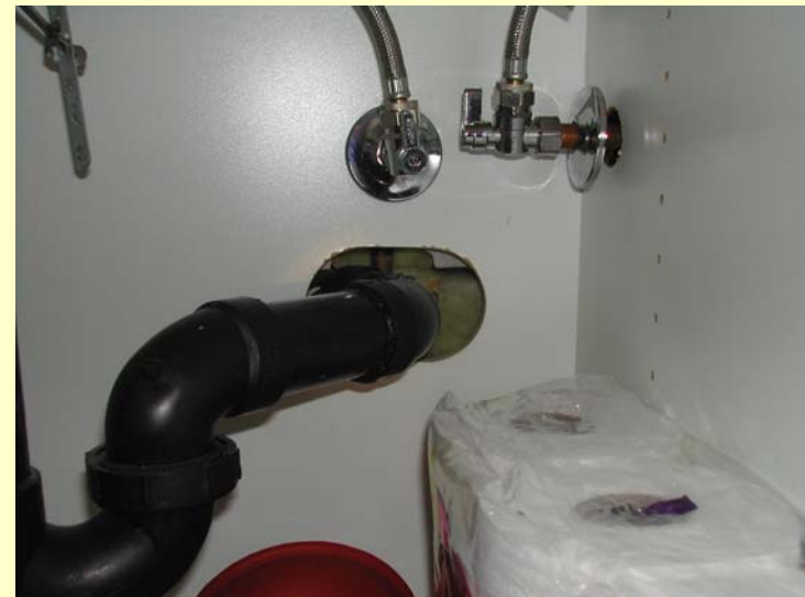
Wall holes around plumbing lines in Homes A & F
