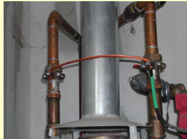
Uninsulated pipes in two PV homes
