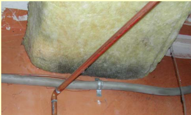
Dark banding indicates area of duct air leakage in 2 PV homes.
