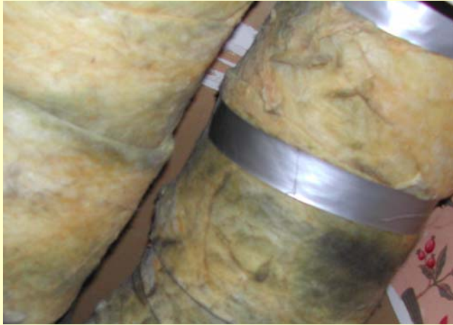
Dark banding indicates area of duct air leakage in 2 PV homes.
