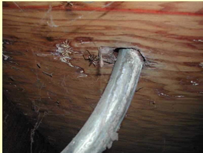
Holes around wire and pipe penetrations from crawl space in 2 PV homes
