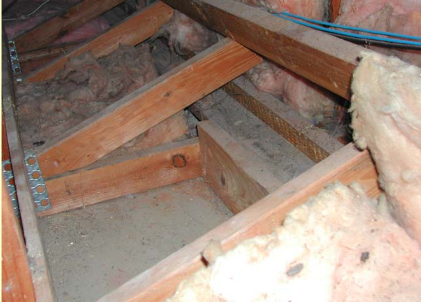
Missing attic insulation in Home A
