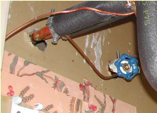
Wall holes around plumbing lines in Homes A & F
