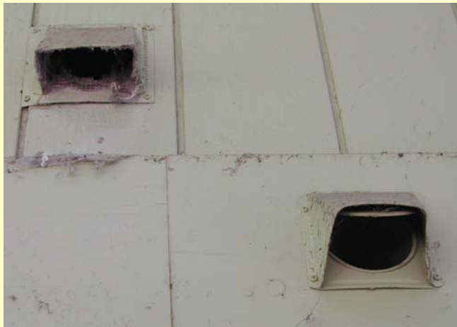
Gravity flappers not closing, House A
